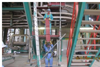
Right Method (standing below scaffolding platform)
