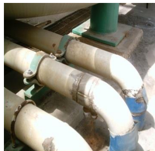
Water entered from the grinding machine vent point
