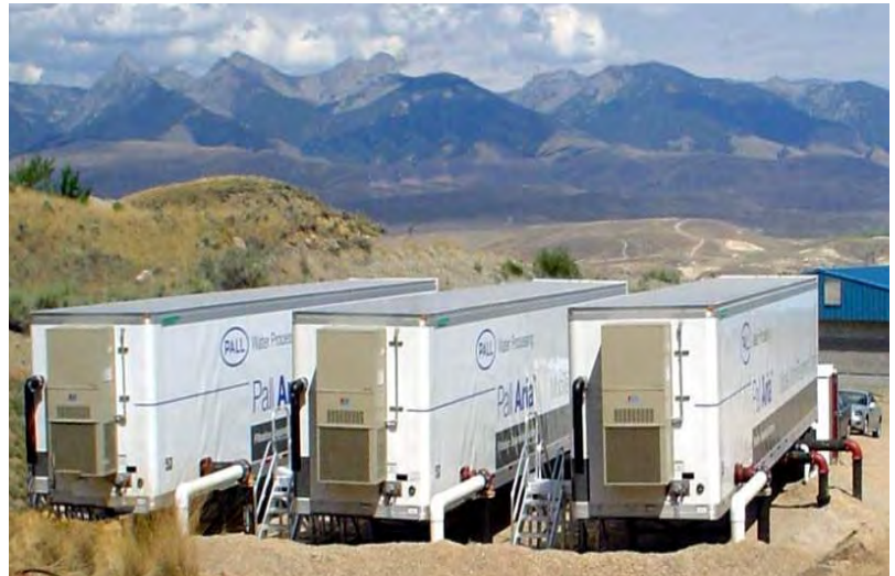
Fig8: Membranes containerized mobile systems
