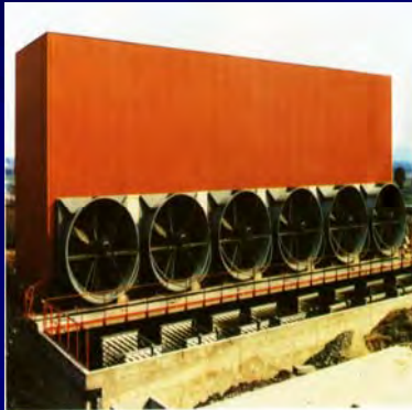
Forced draft – cooling tower – counter flow
