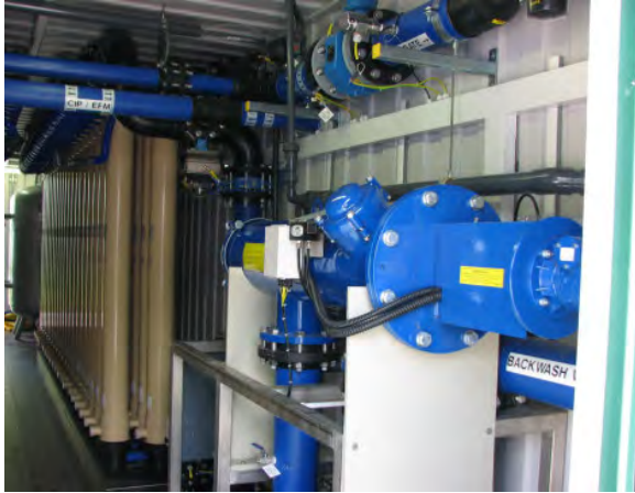
Figure 4a. Large flow Container Up to 6000 m 3 /d
