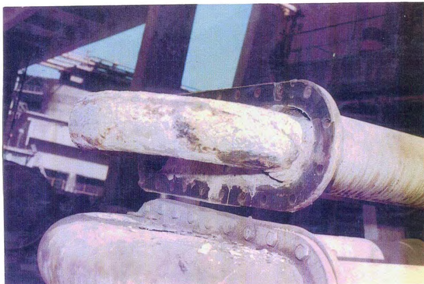
Photo of fouled inter-cooler
