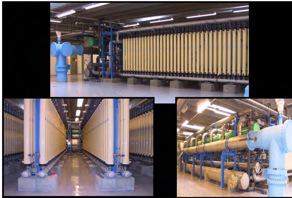
Figure 3: Custom-Designed System for 25 ML/d Capacity with 4 trains
