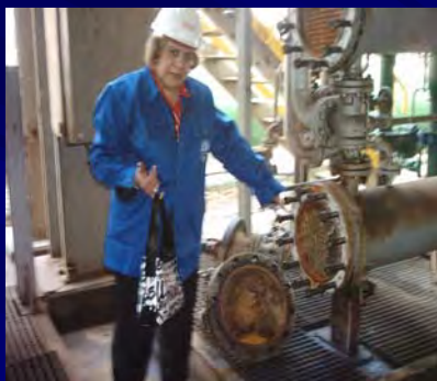
Inter stage cooler of CO 2 compressor
