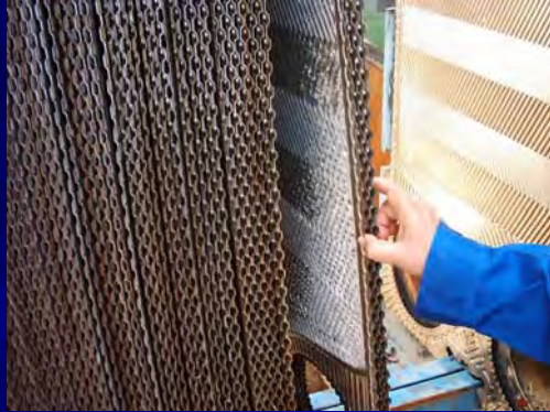
Plate cooler in Nitric Acid plant having heavy scales of Calcium Phosphate and Calcium carbonate
