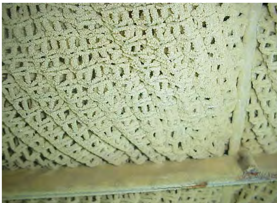
Figure (4). Demister of stage No: 6
