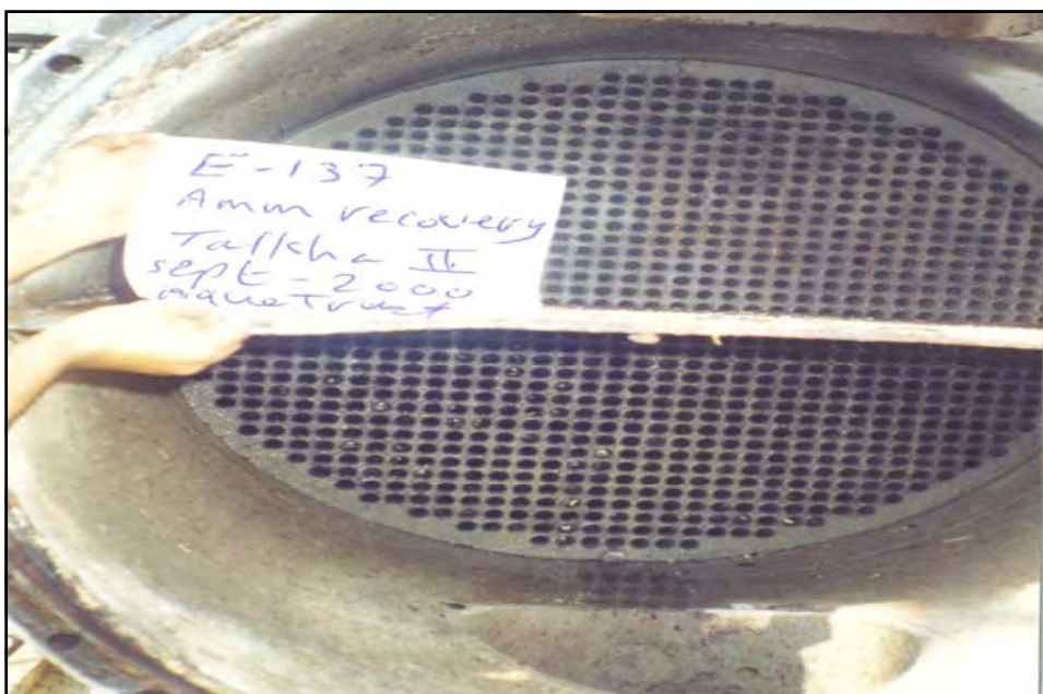
Clean heat exchanger after receiving the above mentioned program at Delta fertilizer – Talkha II – Ammonia plant
