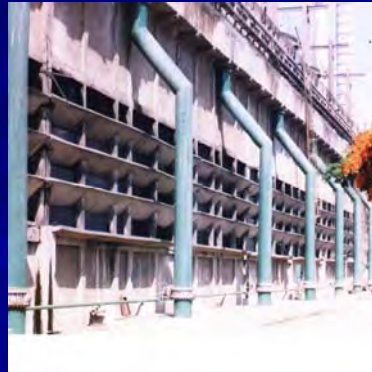
Ammonia plant cooling tower – counter flow
