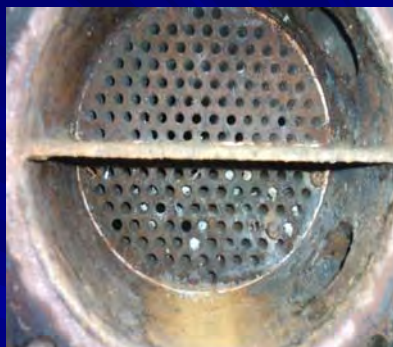
Oil cooler of compressor
