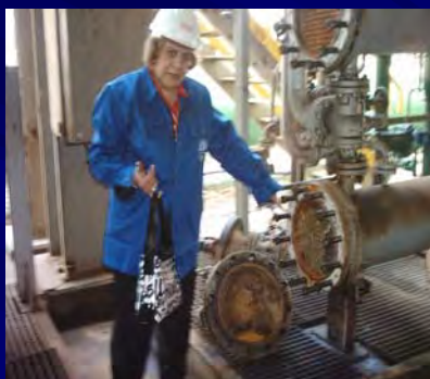
Inter stage cooler of CO 2 compressor
