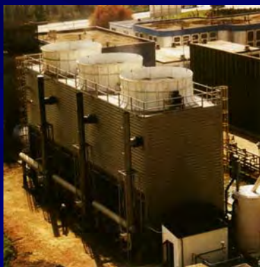
Induced draft – counter flow
