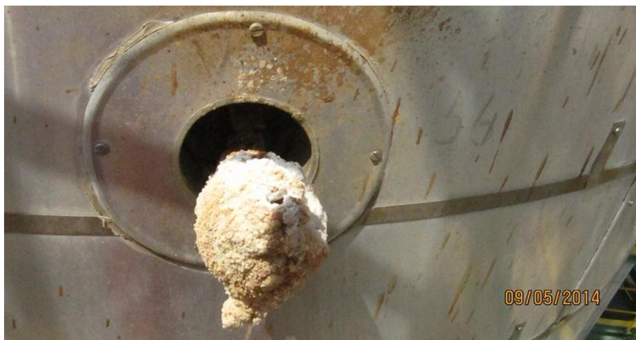
Fig. 3: (Leakage through Weephole)
