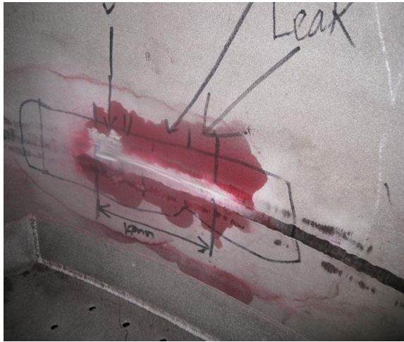
Figs. 9 & 10: (Leakage Area) & (Pinpoint Location)
